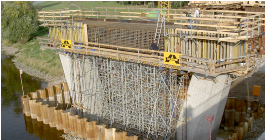
Work under way on the bridge
